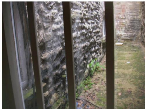
The light-well considered to be promoting damp within the building is itself a remnant from the medieval burgage plot – having originally been an alleyway/snicket/ginnel alongside the building. It has been largely absorbed into the buildings on the site, leaving but a 'light-well' to speak of its former function.
