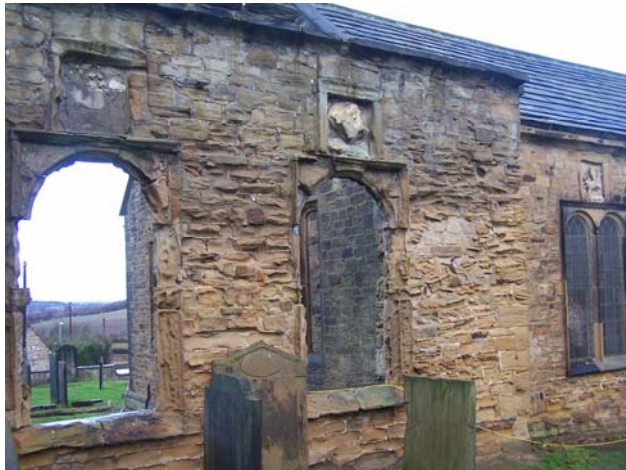
Roofless wall, Holy Trinity Church Wentworth village
